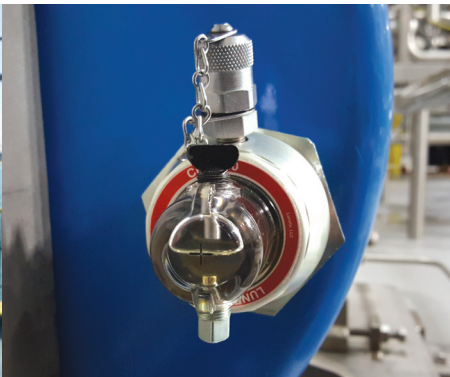
Screw Pump - Bottling Plant
